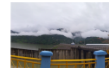
a) Thoubal Multipurpose project
